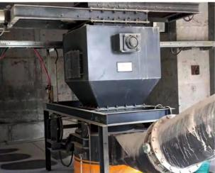
After the loaded truck is parked, the loading personnel press the telescopic tube lowering button on site, and the telescopic tube will drop to the position or stop where it needs to be lowered. The personnel in the central control room or on-site personnel are given the command to open the gate, and the personnel in the central control room pre-set the opening of the gate (4~20mA).
